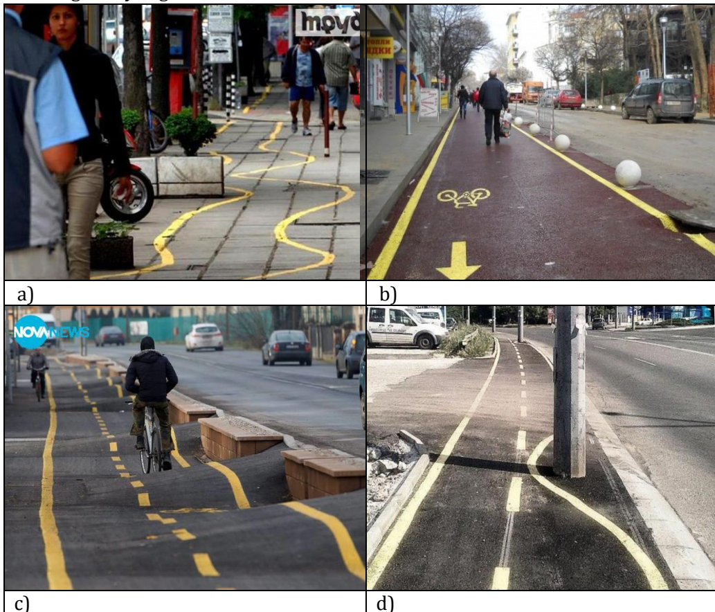
Figure 2. Pictures from articles about failures in the design for the bikeways in Sofia, Varna and Burgas.
